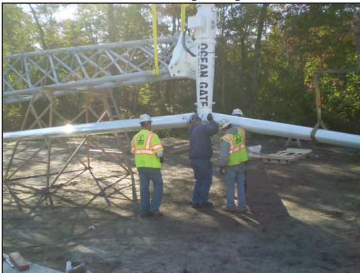
Personnel are pictured attaching blades to the tower.
