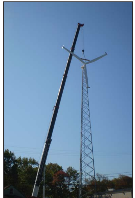
Final erection of the 120 feet tall tower.
