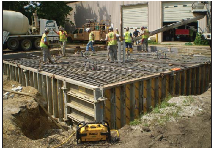
Creamer personnel are pictured constructing the foundation for the wind turbine.
