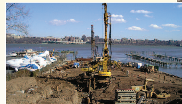
Drilling and installing piles
