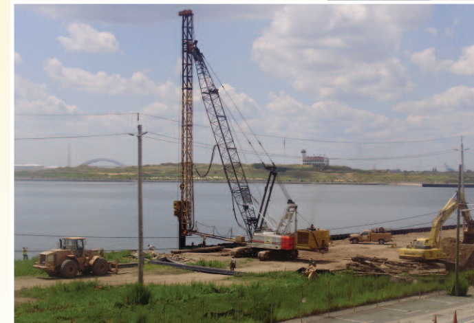
Bulkhead Installation
